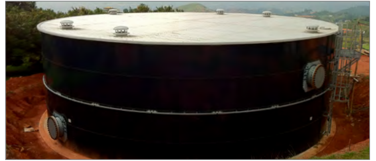
Trough Deck Roof – Drinking Water
