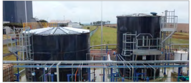
Tapered Beam Roof – Brazil
